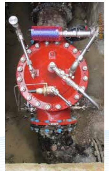
Electronics field retrofit and commissioning
